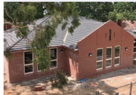
Larritt House during building works.
